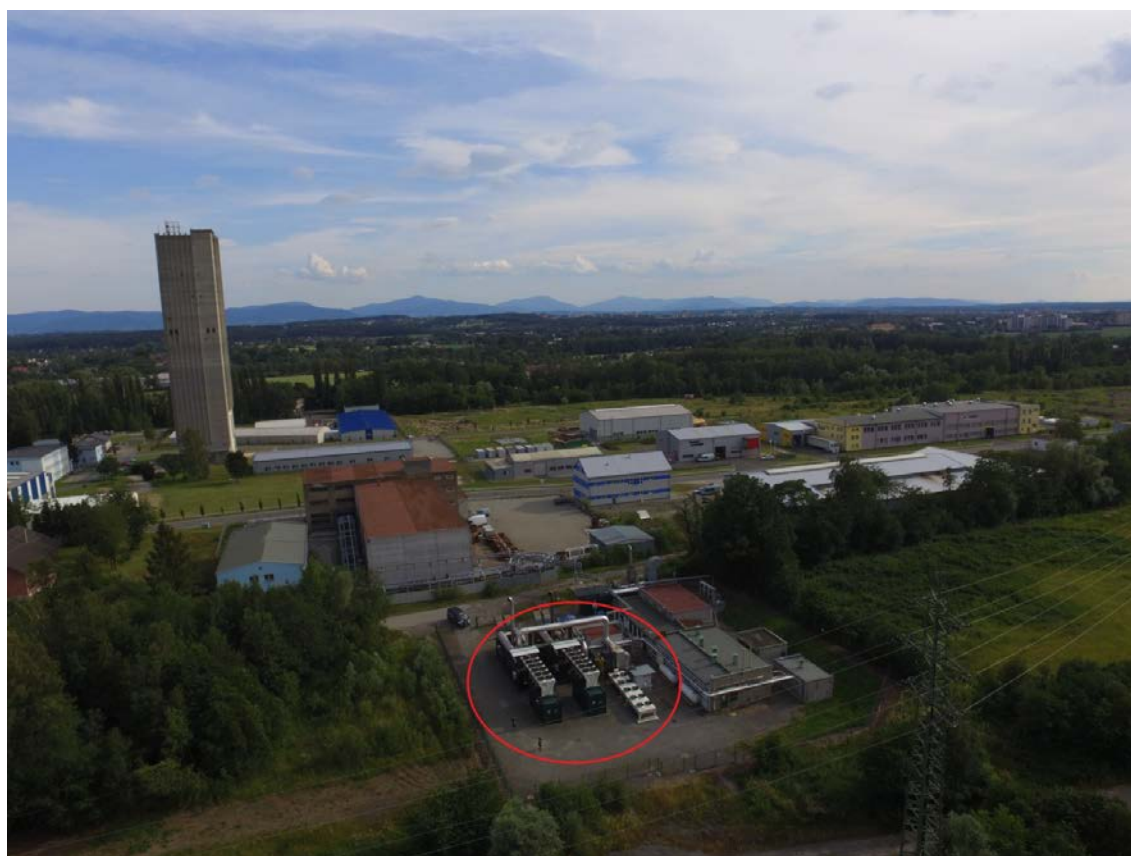
Fig. 2. Cogeneration units on the brownfield (a former mine František) (Source: own)
